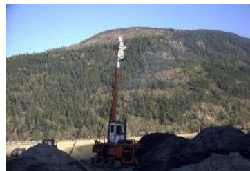
Dragline after the Device was installed
